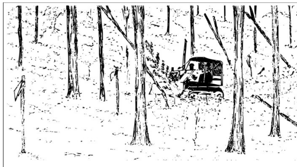
Figure 50 Bulldozer follows flagged alignment in the forest.
